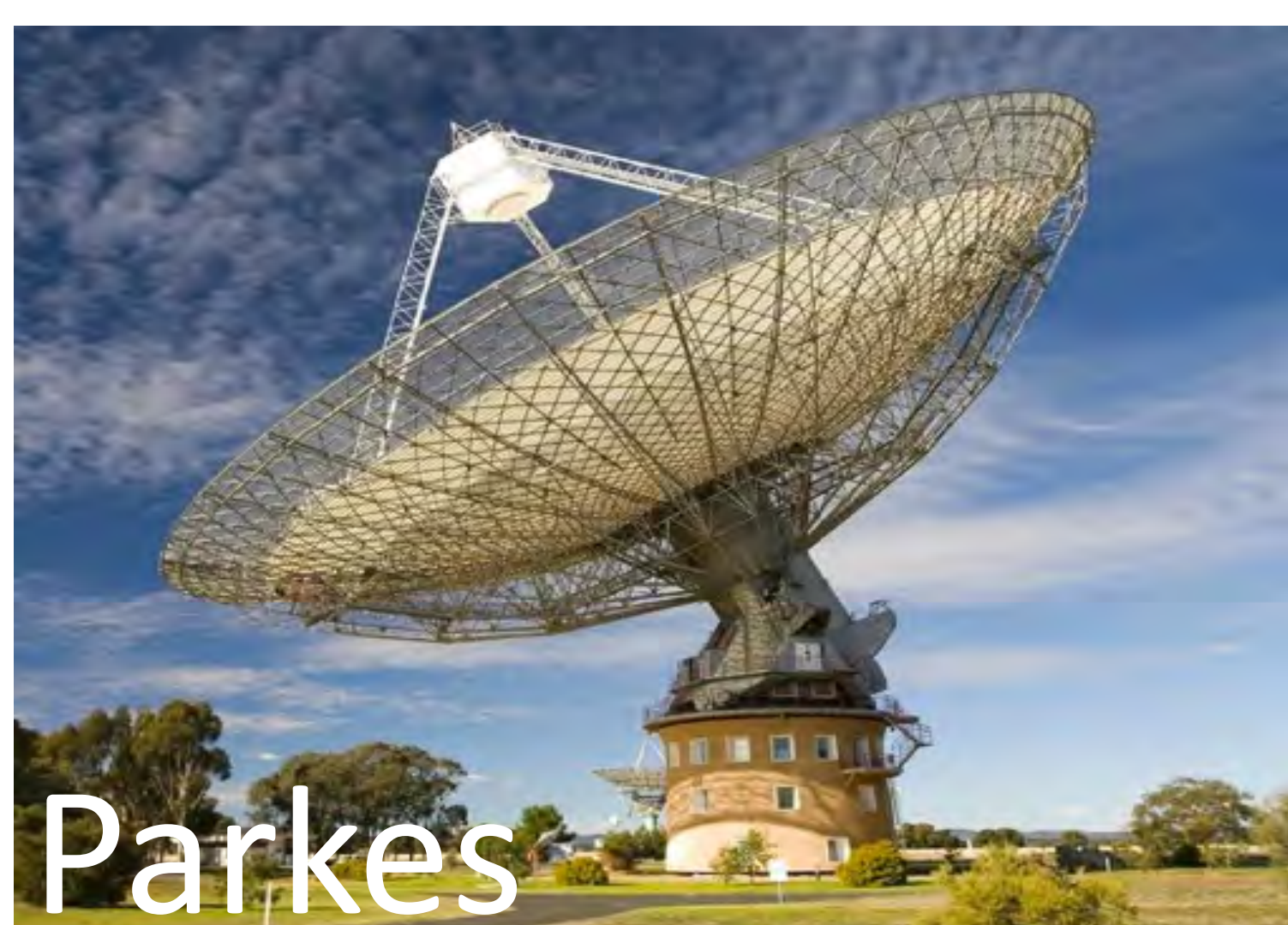
Figure 1: Parkes Telescope (The Dish) is located in New South Wales Australia. It operates at 700 – 4000MHz and offers 3300MHz bandwidth.
